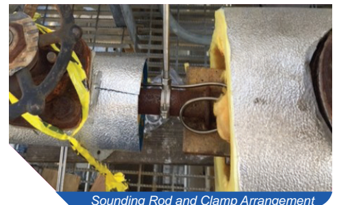
Sounding Rod and Clamp Arrangement
