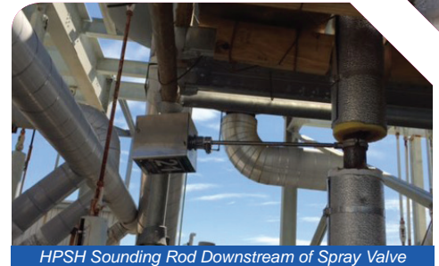
HPSH Sounding Rod Downstream of Spray Valve
