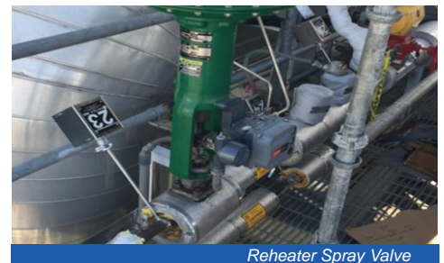
Reheater Spray Valve
